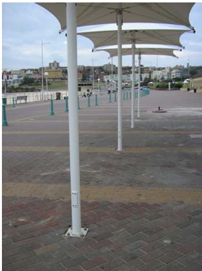
Nick's Café – Bolt plate set into promenade and secured with bolts – These bolts require bolt threads cemented into concrete and the tops tightened – Permanent .
