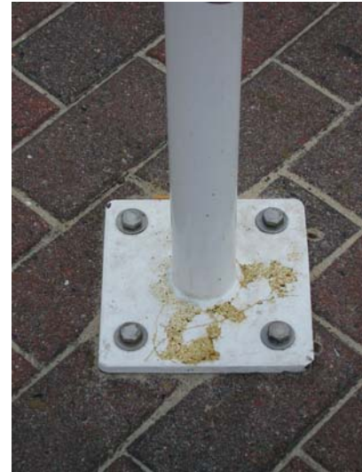
Lusher's Bar Gelato – Bolt plate sitting above promenade with bolts screwed into the promenade – Temporary .
