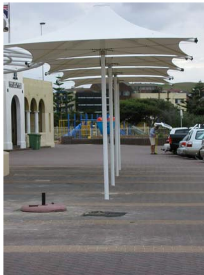
Nick's Café – Bolt plate set into promenade and secured with bolts – These bolts require bolt threads cemented into concrete and the tops tightened – Permanent .
