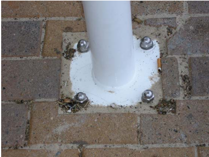
Nick's Café – Bolt plate set into promenade and secured with bolts – These bolts require bolt threads cemented into concrete and the tops tightened – Permanent .
